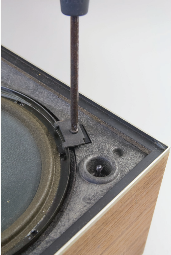
Re-mount the woofer with the respective brackets.
